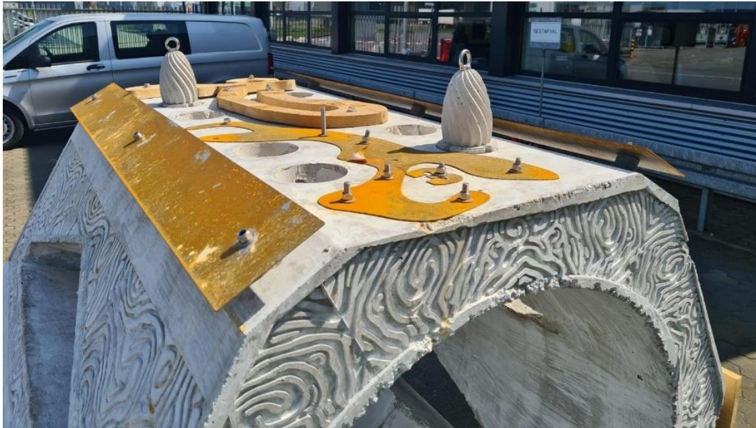
Figure 3. Close up of some of the ExoLodge wood and metal features and removable reef plugs.
