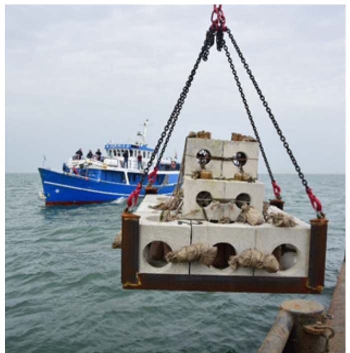
Figure 21 & 22: A reef dome and reef blocks (photos: De Rijke Noordzee).
