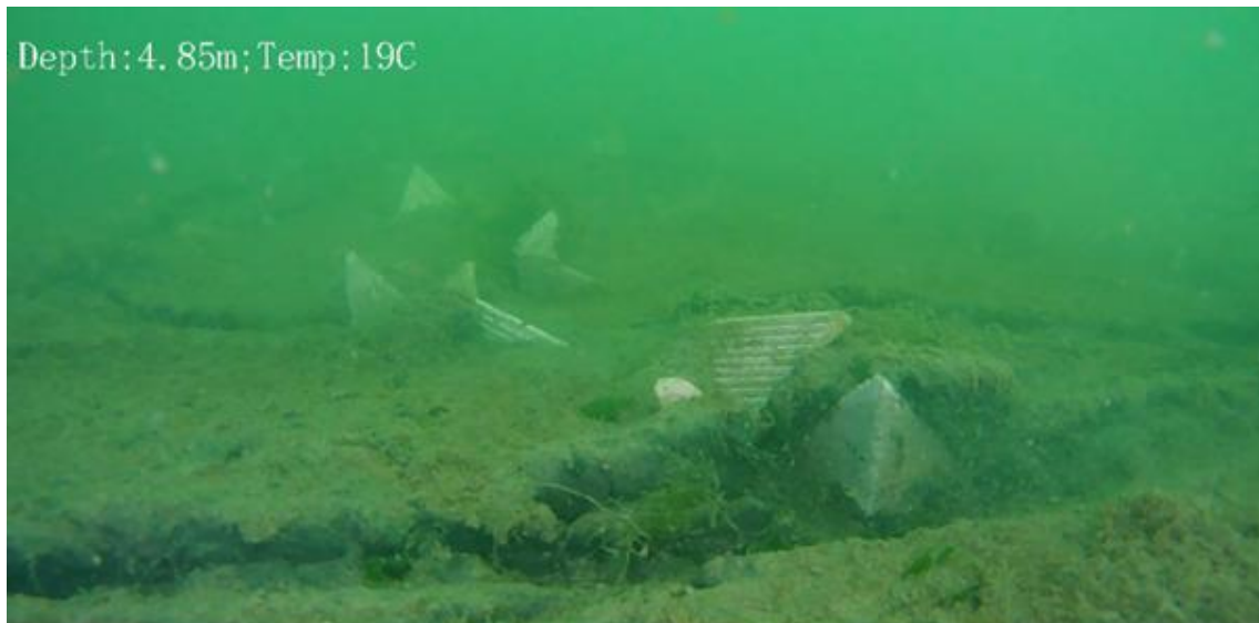
FIGURE 24. ROV OBSERVING OF THE REEFBOOSTERS IN PLOT 1 RIGHT AFTER DEPLOYMENT.
